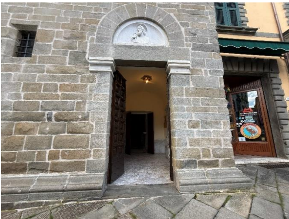
16 Side church entrance
